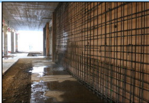
Shear wall reinforcement, above, and construction of the gym building foundations and attachment point to old library wall, right.
