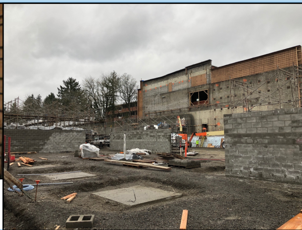
Shear wall reinforcement, above, and construction of the gym building foundations and attachment point to old library wall, right.
